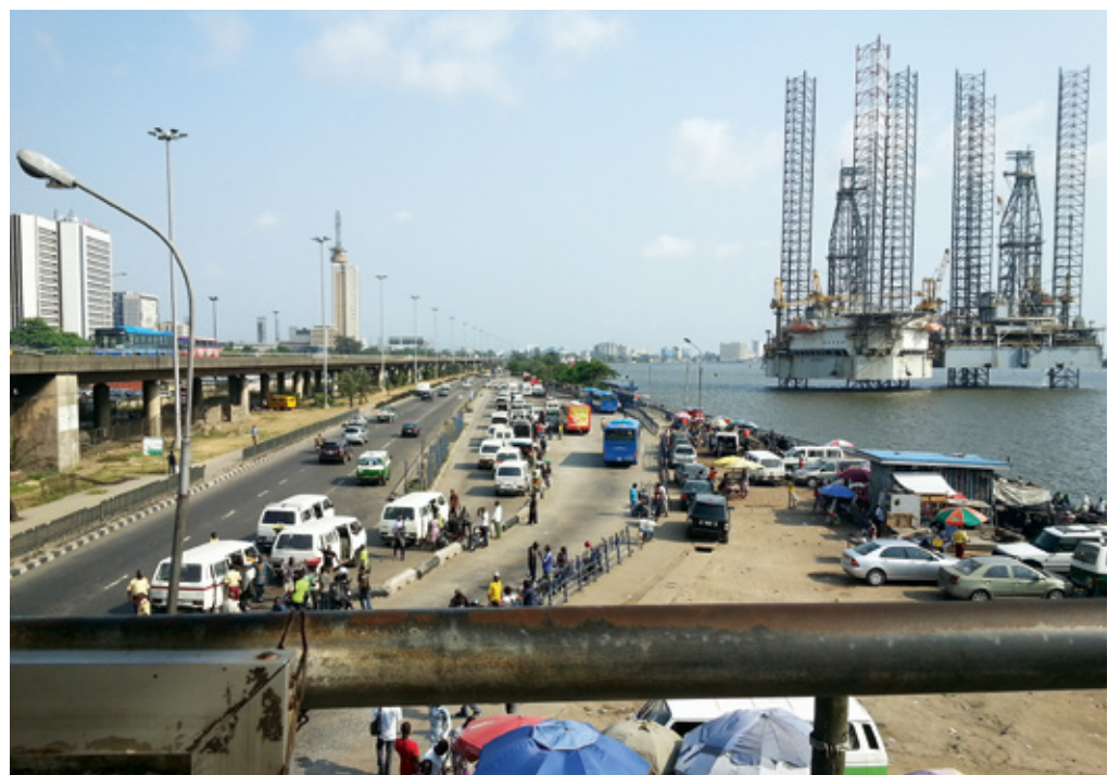
Lagos Island Downtown Ring Road Bus Stop
